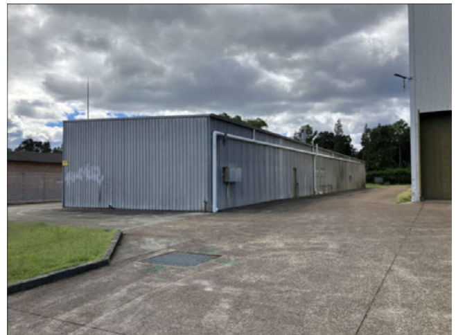
Figure 18 – Concrete driveways, and evidence of extensive underground stormwater infrastructure
