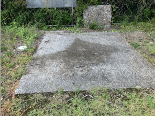
Figure 21 – Evidence of previous underground services on the site
